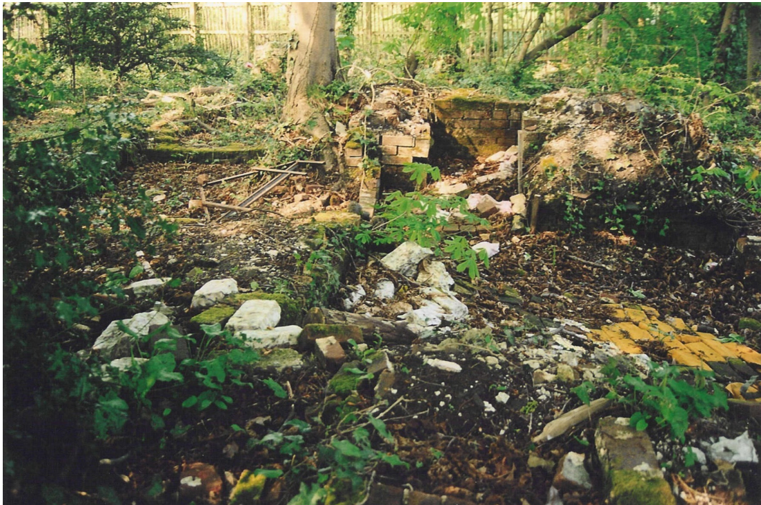
Plate 4: Remains of the North Lodge, from the South
