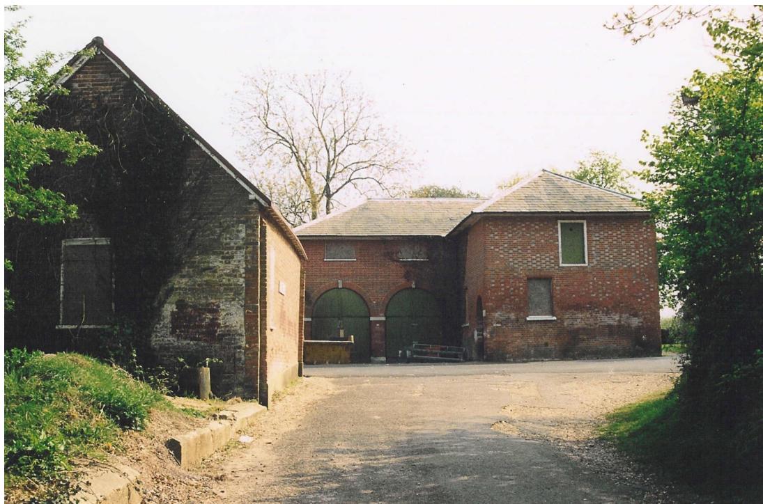
Plate 5 : The former stable block from the North West
